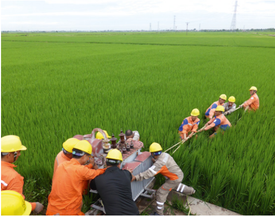
Vietnam Electricity workers remove an old transformer to make way for one of higher capacity. (Photo: Thi Phuong Thao Vu, 2019)
